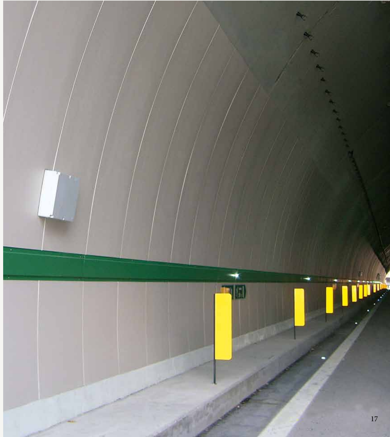
2008 Tunnel Autostradale Bologna-Firenze - Italia Bologna-Florence Motorway Tunnel - Italy LAMINAM 3+ Collection Avorio 1000x3000
